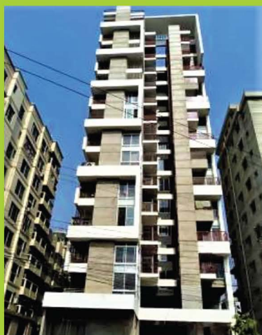
KDS Properties Ltd. Automatic Fire Hydrant System.
