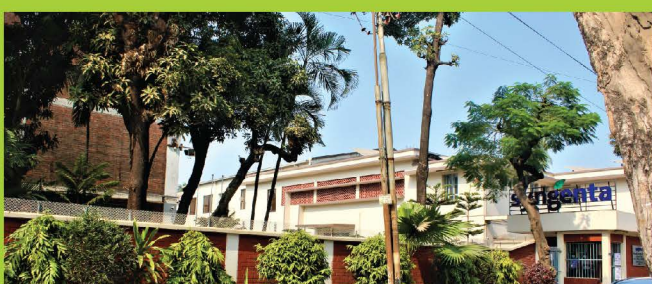
Syngenta BD Ltd. Civil Construction & Fire, Electrical System
