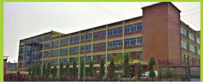
Park (Bangladesh) Company Ltd. Automatic Fire Hydrant System.
