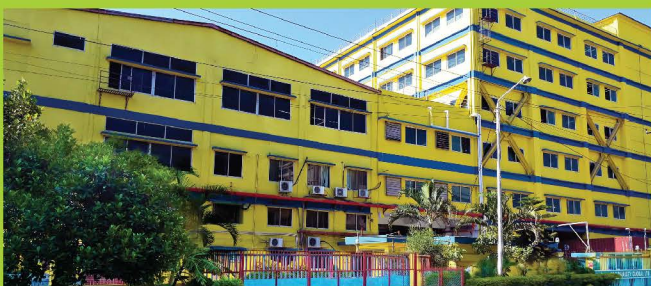
Campvalley Global Ltd-Unit-1. Automatic Fire Hydrant & Sprinkler System.
