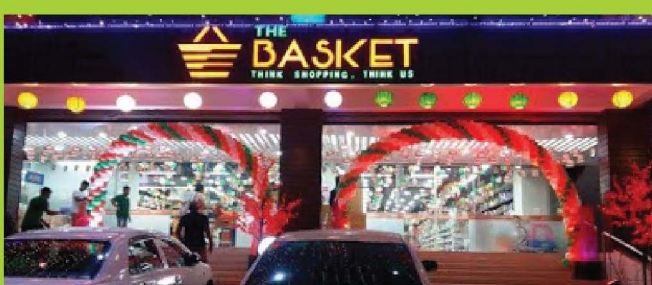
The Basket. Automatic Fire Detection & Alarm System.
