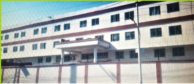
New Era Fashions Mfrs (BD) Ltd. Automatic Fire Detection & Alarm System & Fire Door UL Listed
