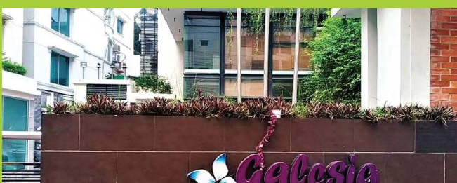
Galesia Hotel & Resort Ltd. Automatic Fire Alarm & Detection System.
