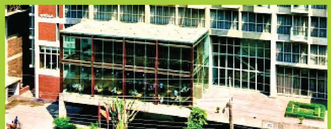
Grand Heritage Ltd. Total Electrical, Booster Pump, Plumbing Solutions.
