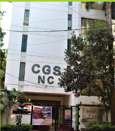
Finlay Properties Ltd-CGS-NC. Automatic Fire Hydrant & Sprinkler System, Fire Detection & Alarm System, Fire Door System & Fire Extinguisher System.
