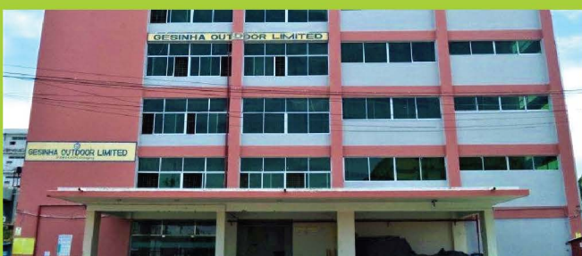
Gesinha Outdoor Ltd. Automatic Fire Hydrant System & Fire Detection & Alarm System.
