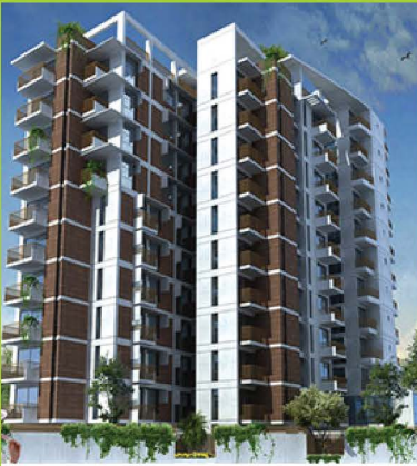
ANZ Properties Ltd-S.M Moon Yard. Automatic Fire Hydrant & Sprinkler System, Fire Detection & Alarm System, Public Addressable System, Fire Door System & Fire Extinguisher.
