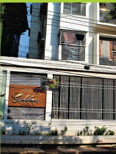
CPDL-Gulshan Grove. Automatic Fire Hydrant System.
