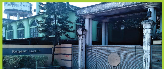
Habib Group-Regent Textile Mills Ltd. Automatic Fire Detection & Alarm System & Fire Rated Glass Door-UL Listed.
