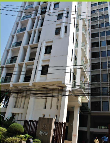
Concord-Alpona. Automatic Fire Hydrant & Sprinkler System, Fire Detection & Alarm System.
