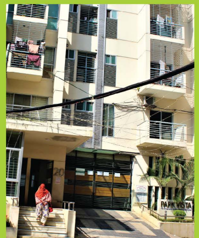
Park Bista Automatic Fire Hydrant System & Fire Door.
