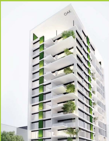
Ranks White Oak Automatic Fire Hydrant & Sprinkler System, Fire Detection & Alarm System, Fire Door & PA System.
