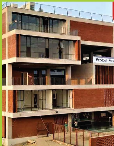
Frobel Academy School-BSRM. Automatic Fire Hydrant & Sprinkler System, Fire Detection & Alarm System, Fire Door & Fire Extinguisher
