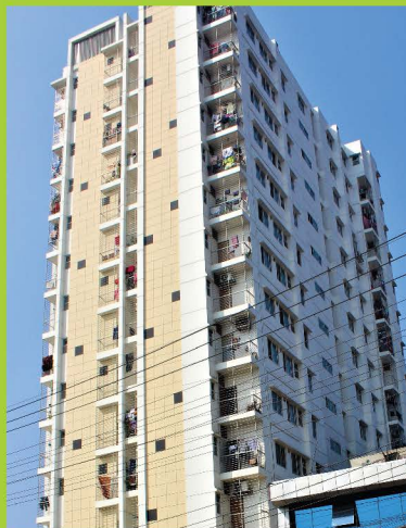
Jumaira Holding Ltd-Bahamas. Automatic Fire Hydrant System.
