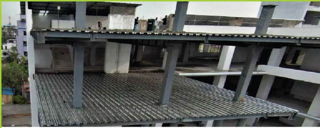
City Corporation - BMDF- World Bank-Commercial Complex. Automatic Fire Hydrant & Sprinkler System, Fire Detection & Alarm System, Public Addressable System, Fire Door System
