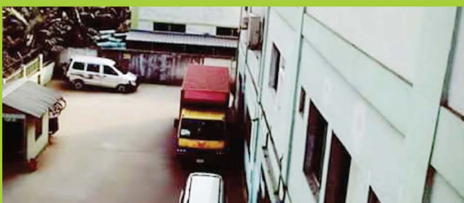
Bestec (BD) Limited. Automatic Fire Detection & Alarm System.
