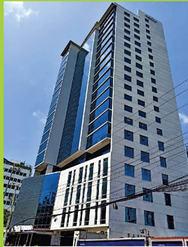
Four H Group-Aerial Properties Ltd-Legend. Automatic Fire Hydrant & Sprinkler System, Fire Detection & Alarm System, Fire Door System & Fire Extinguisher System.
