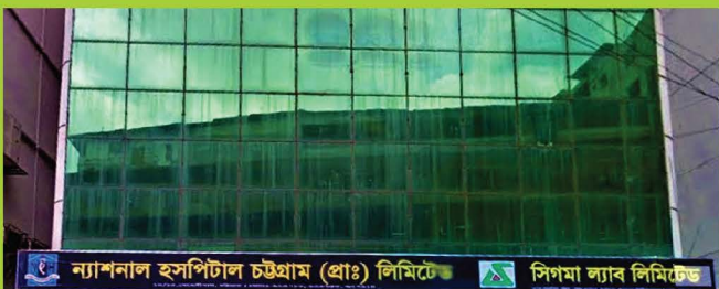
National Hospital. Automatic Fire Hydrant System.
