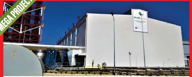
Feni Lanka Power Plant. Fire Suppression System-NAF S125BOC FS125 Gas, UL Listed & Automatic Fire Hydrant Accessories.
