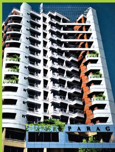
CPDL-Paragon City. Automatic Fire Hydrant System.
