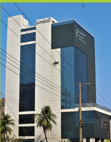
Jumaira Holding Ltd-Project-Fairmont Trade Center. Automatic Fire Hydrant & Sprinkler System.
