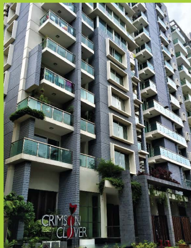
CPDL-Crimson Clover. Automatic Fire Hydrant & Fire Door System
