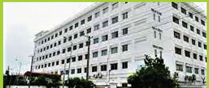
Hong Kong Denim (Pvt.) Limited. Automatic Fire Detection & Alarm System.
