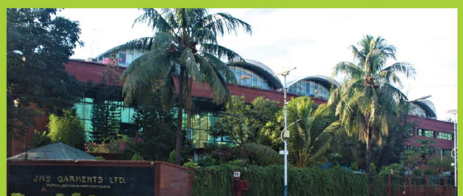
JMS GROUP. Automatic Fire Hydrant & Sprinkler System, Fire Detection & Alarm System.
