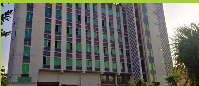
Al-Ittefaq Textiles Ltd. Automatic Fire Hydrant & Sprinkler System & Fire Detection & Alarm System.
