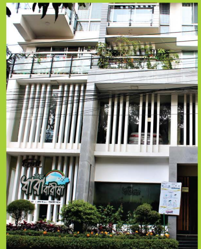
CPDL-Dara Barisha. Automatic Fire Hydrant System.
