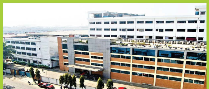
Sea Tex Ltd & Sea Blue Textile Ltd. Automatic Fire Hydrant System & Fire Detection & Alarm System.
