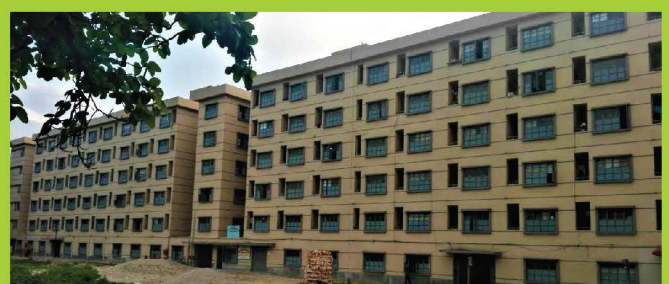
M.M. Ispahani Group-Dormitory Building. Automatic Fire Hydrant System.
