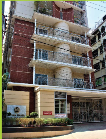
Bti-Sater Manzil. Automatic Fire Hydrant System.
