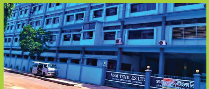
MZM Textile Ltd. Automatic Fire Hydrant System.
