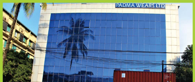
Padma Wears Ltd. Automatic Fire Hydrant System & Fire Detection & Alarm System.
