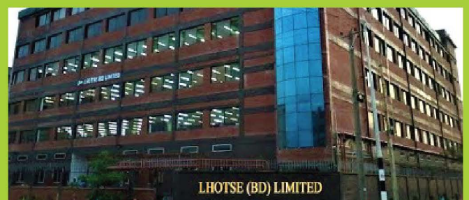
Lhotse (BD) Limited. Automatic Fire Hydrant System.
