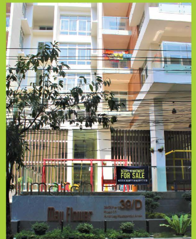
Jumaira Holding Ltd-May Flower. Automatic Fire Hydrant System.
