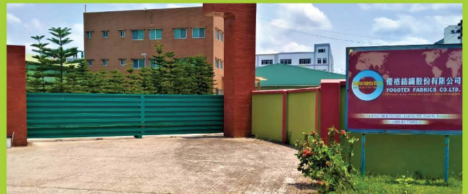
Yogatex Fabries Co. Ltd. Automatic Fire Hydrant System.
