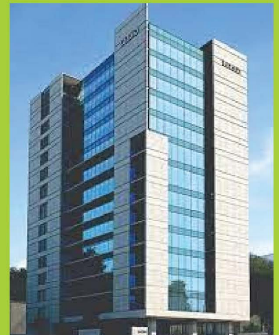
Labaid Cancer Hospital Dhaka Automatic Fire Hydrant & Sprinkler System, Fire Detection & Alarm System, Fire Door UL Listed.
