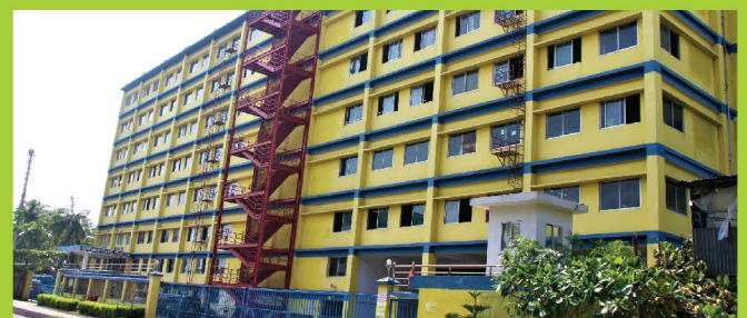
Campvalley Global Ltd-Unit-2. Automatic Fire Hydrant & Sprinkler System.
