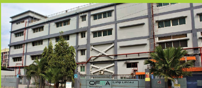
OFMA Camp Limited. Automatic Fire Hydrant System & Fire Detection & Alarm System.
